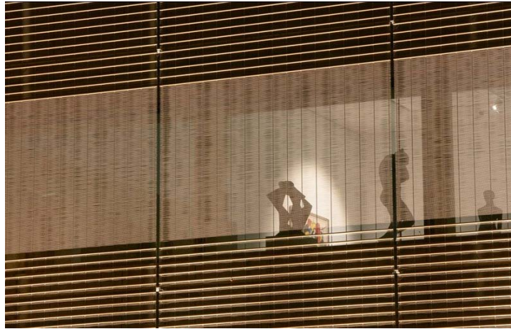
Picture 6-8: The stainless steel fabric from GKD shows a significantly higher degree of transparency in front of the large-format glazed surfaces than in front of the fiber cement panels.
