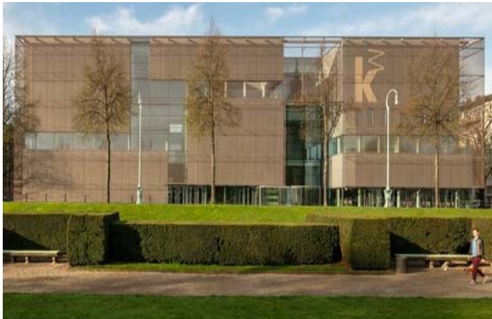
Picture 1: A shell made of bronze-colored stainless steel fabric from GKD characterizes the new façade of the Kunsthalle Mannheim.
