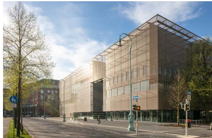
Picture 2: The varying transparency of the fabric from GKD translates the scale of the building, creating a balanced sense of near and far.
