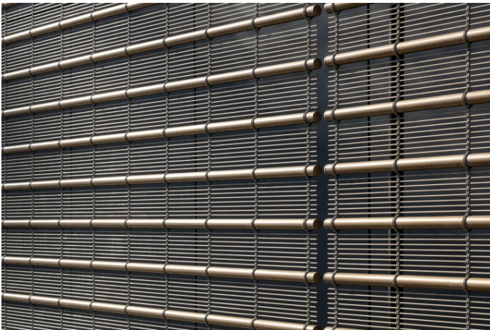
Picture 9-10: GKD wove stainless steel wires and tubes of 3 mm and 25 mm into four-wire warp wire groups made of untreated stainless steel.
