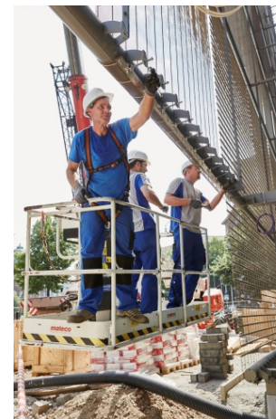
Picture 14-15: The installation of the GKD-fabric-panels measuring around 20 meters in length and 3.3 meters in width was precision work.
