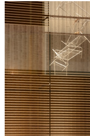
Picture 6-8: The stainless steel fabric from GKD shows a significantly higher degree of transparency in front of the large-format glazed surfaces than in front of the fiber cement panels.
