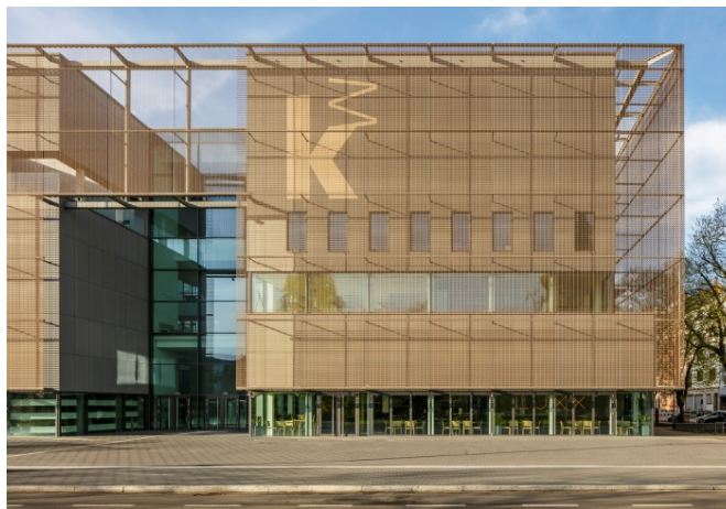
Picture 3-4: The fabric design developed by GKD especially for the Kunsthalle Mannheim made of bronze-colored cables, wires and tubes builds a sophisticated membran in front of the huge building.
