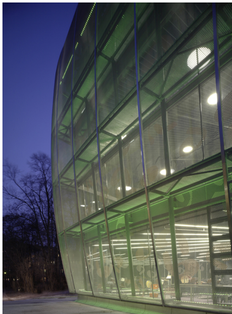
Picture 3: At night, LEDs transform the protective membrane into a fusion of transparency and colours.
