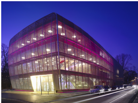
Picture 2: 66 panels of GKD Omega mesh make up the 4,000 square meter translucent skin.
